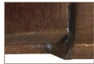
Showing an exposed board at breadboard joint
