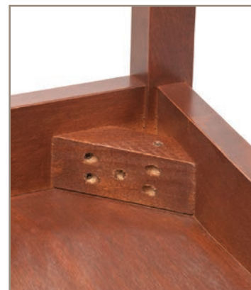
Corner block strengthens corners
