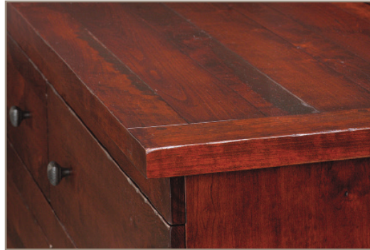
Showing an exposed groove in breadboard
