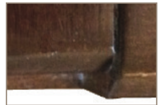
Showing an exposed board at breadboard joint
