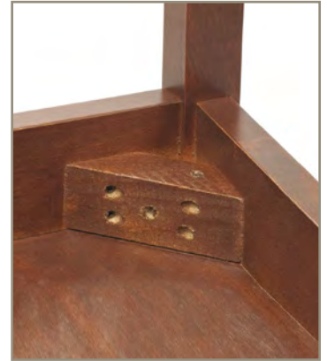
Corner block strengthens corners
